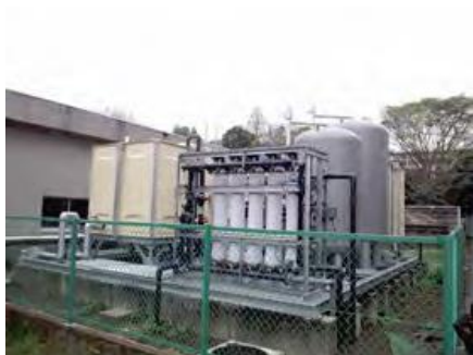
Photo: underground water purification system
